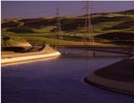
SOURCE WATER PUMPING
