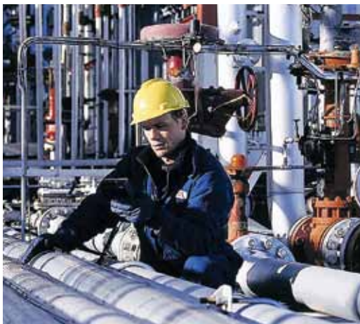
Natural Gas Pipe Line Worker
